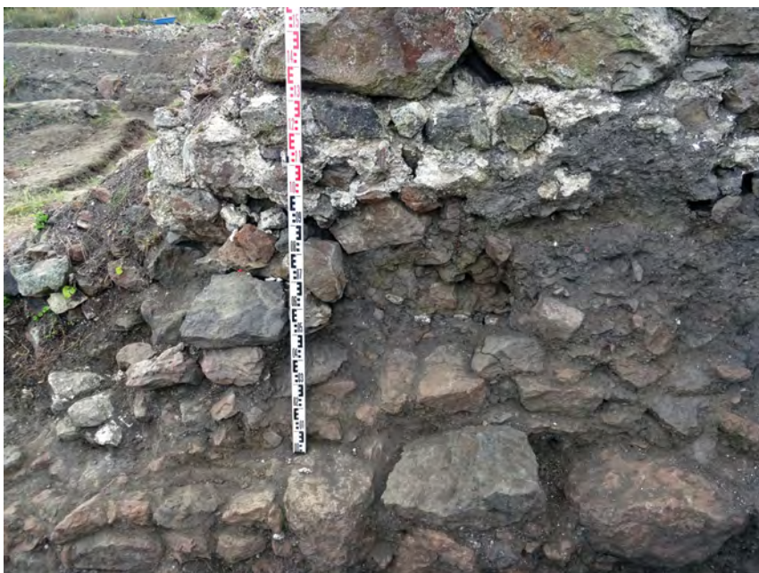
Fig. 26, fig. 27 – The west wall of the passage, external face, resting on a layer of stones and yellow clay piled on top of the early Byzantine wall with mud binder
