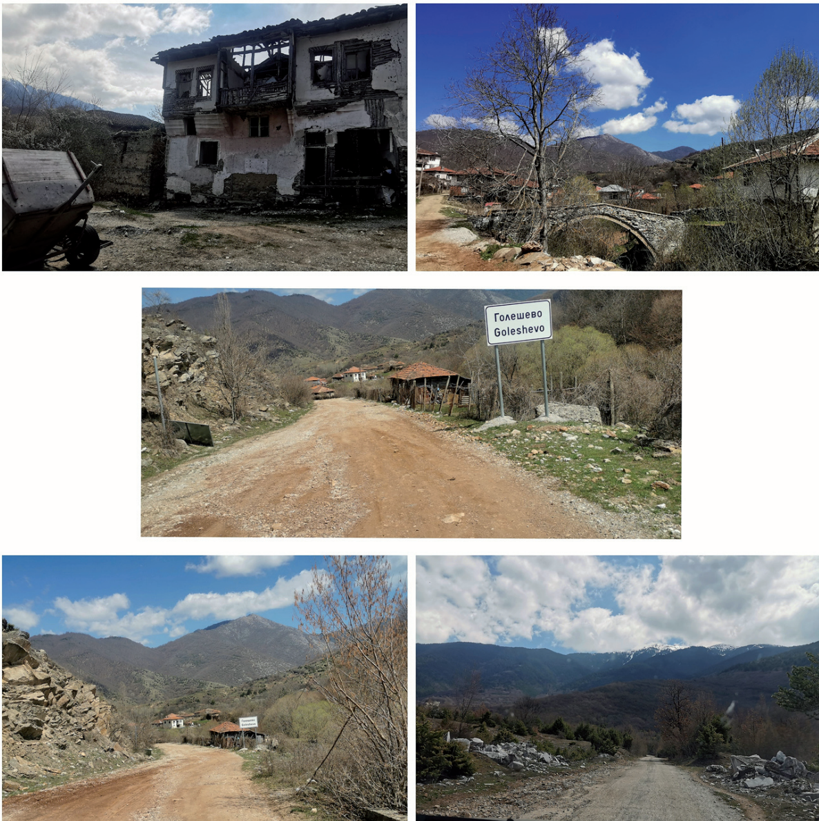
Illustration 7. The infrastructure leading to the Goleshovo village, along with the village sign and views from its centre.
